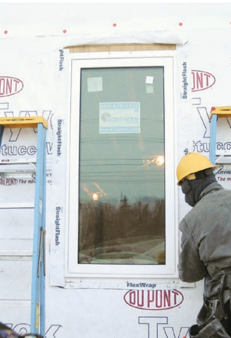
Figure 1. In a REMOTE wall, the sheathing is covered with a barrier membrane — either peel-and-stick (top), 6-mil polyethylene sheeting (above), or, in wet climates or beneath EIFS cladding, a wrinkled drainage material such as StuccoWrap (left). Installed before the roof is framed, the barrier membrane extends over the top plates and is later sealed to the poly air barrier on the ceiling of the house's top floor.
