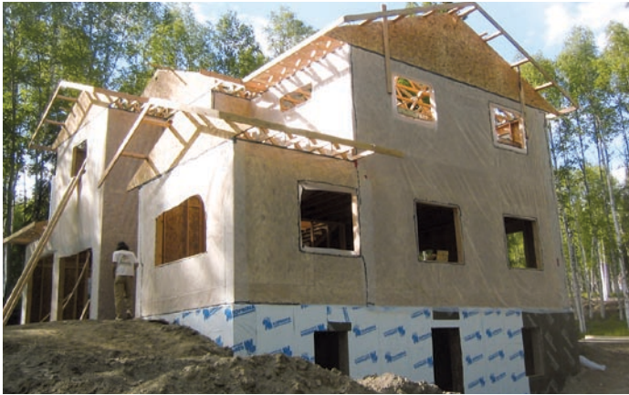
Figure 1. In a REMOTE wall, the sheathing is covered with a barrier membrane — either peel-and-stick (top), 6-mil polyethylene sheeting (above), or, in wet climates or beneath EIFS cladding, a wrinkled drainage material such as StuccoWrap (left). Installed before the roof is framed, the barrier membrane extends over the top plates and is later sealed to the poly air barrier on the ceiling of the house's top floor.
