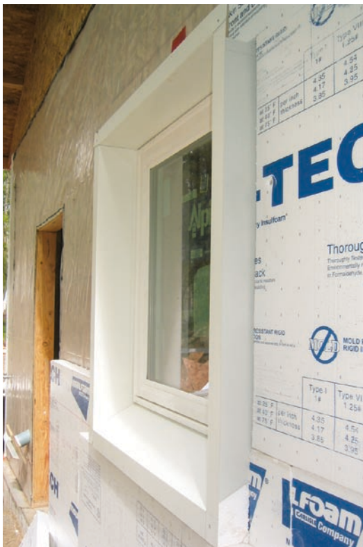
Figure 3. When installing recessed windows, the author uses sill and jamb extensions bent from coated sheet metal. The flanges at the outer edges (left) are carefully placed to allow for the thickness of the foam, \frac{3}{4} -inch strapping, and the vinyl siding, which will tuck underneath. Note the lines of black acoustical caulk used to seal the jamb extensions to the poly membrane and the poly seams (above).
