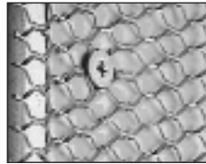
Wire lath to steel or wood studs.
