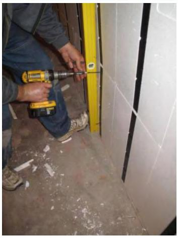
Work your way up the wall. Follow the level using it as a guide and install additional "shim screws" directly above the previous "shim screws" where needed to level out the wall.
