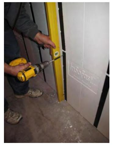
Now deconstruct your wall. Remove all the panels and stack in them in reverse order. (Do not remove the set screws from your panel as they serve as a guide for the amount and type of adhesive that you will apply to your panel.)
