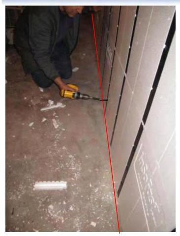
Slowly turn the screw in until the wall is level with the chalk line. Repeat until the entire base of the wall has been trued to the line.
