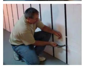
6. Use a hammer to drive the nail into the wall. Don't overdrive the nail. Tap the Perma-grip® fastener until securely seated.
