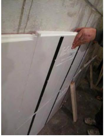
\*We are now placing the panel we cut and carved to fit over the bulge in the wall. Place a continuous bead of glue over the area where the stud was removed.
