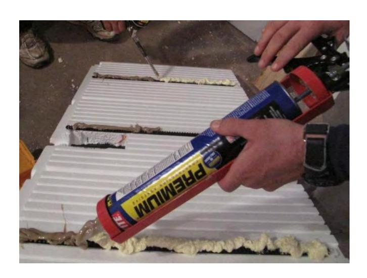
Now you are ready to reassemble your plumb and level wall. Apply a bead of spray foam adhesive to the floor. This will lock the panel in place along that bottom edge.
