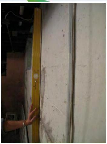
In this photo to the left, if we ignored the bubble and fit our straight edge flush to the top of the wall, the level's straight edge has kicked away from the wall by over 2 ½" at the floor.
