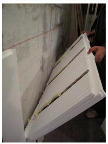
Note the 2 different adhesives being used to provide proper glue contact to secure the panel to the wall.
