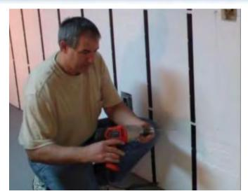
4. Here we will demonstrate installing a Perma-grip® nail. Use a Standard Hammer drill or Rotary Hammer drill to pilot a hole into the concrete wall.
