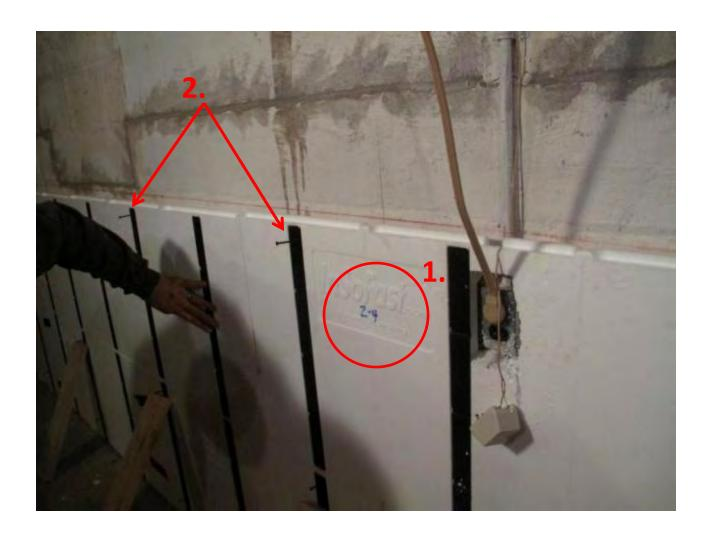
Note that small 2x4s leaning up against the panels keep the panels tight or "braced" to the wall.
