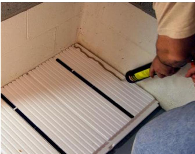
Apply a bead of adhesive directly on the foam on the backside of the InSoFast panel within 2" of corner cut.
