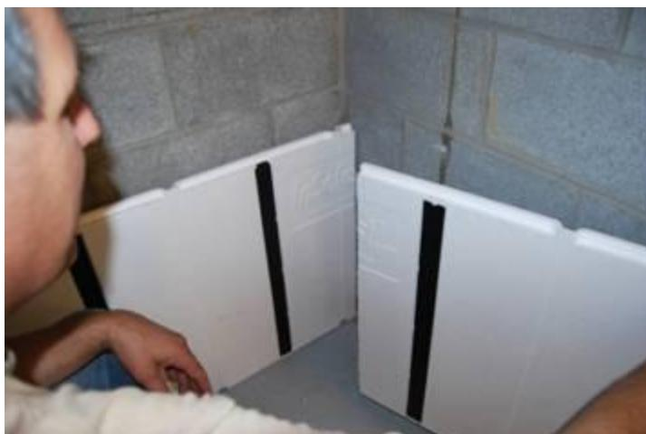
Mark and cut the panels about  $\frac{1}{4}$ " less than actual measurement needed so panels are not tight to the inside or outside corners, leaving a  $\frac{1}{4}$ " gap reduces the push out stress on the panels.
