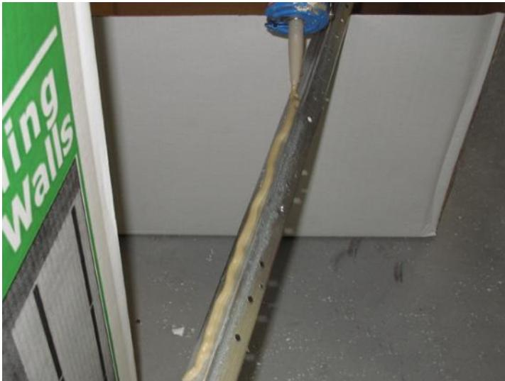
Apply a bead of adhesive directly on to the metal utility corner angle.
