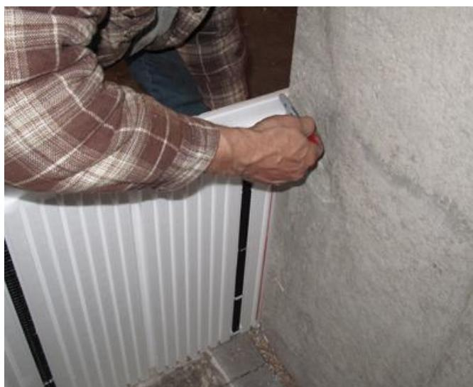
Mark and cut the panels about  $\frac{1}{4}$ " less than actual measurement needed so panels are not tight to the inside or outside corners, leaving a  $\frac{1}{4}$ " gap reduces the push out stress on the panels.
