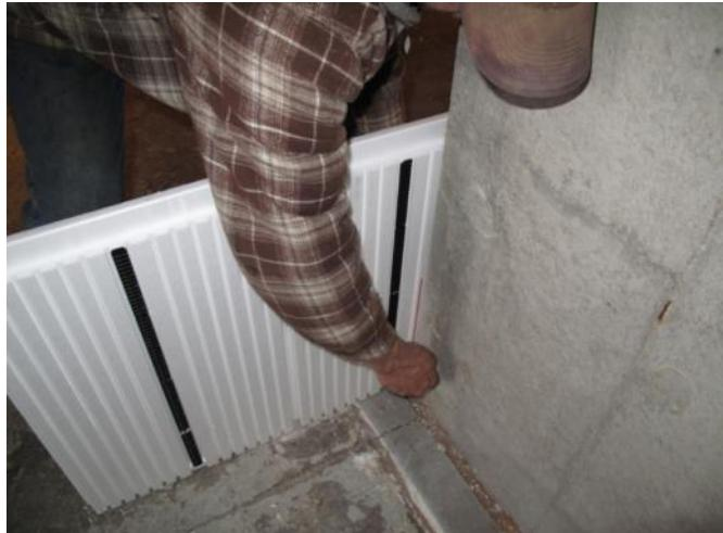
InSoFast is rough framing and not fine carpentry. Cuts should not be tight. You can always go back and fill in any voids or gaps with spray foam
