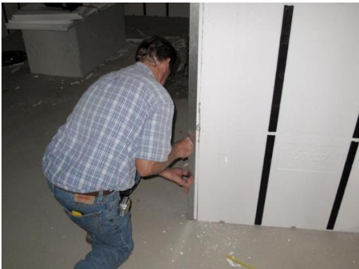
Apply beads of adhesive to the metal "L" angle, press into the corner then duct tape the corner until the glue sets.
