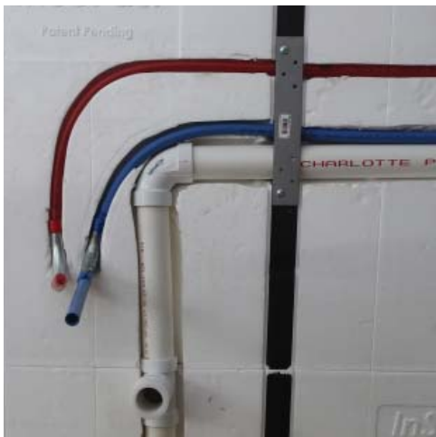
Use protection plates where necessary.
