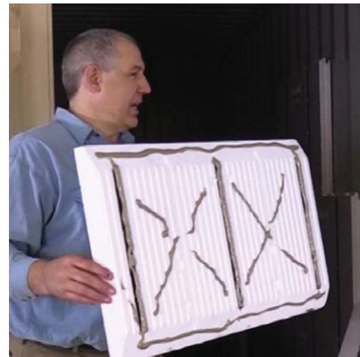
Use plenty of adhesive on the doors.
