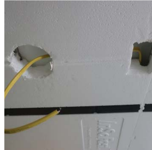
Run wire around the corner.
