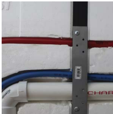
Pex pipe running along side waste.
