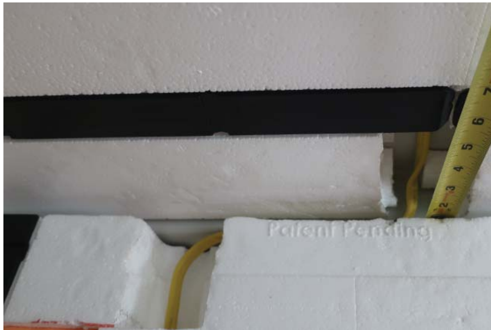
Push with wiring all the way back to the beam.
