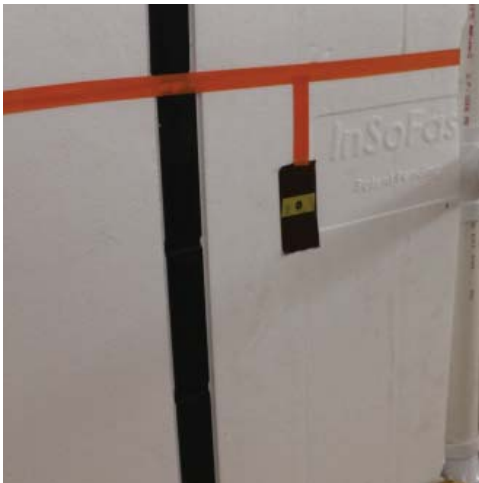
Outlet located below horizontal raceway.
