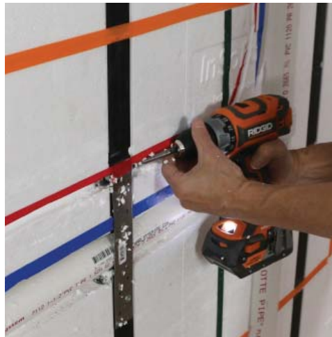
Drill behind the stud for the pex pipe.
