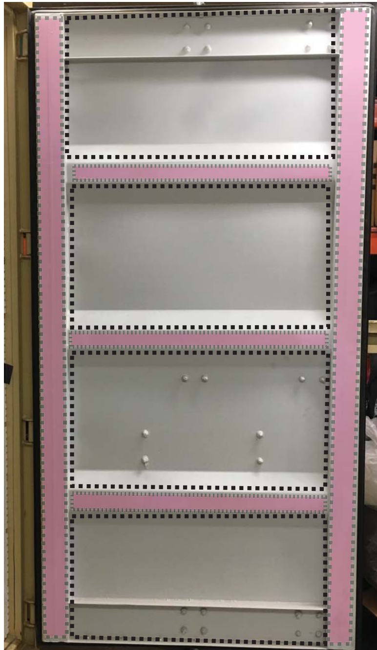
Cutting diagram that illustrates when InSoFast panels and sheet foam is used.
