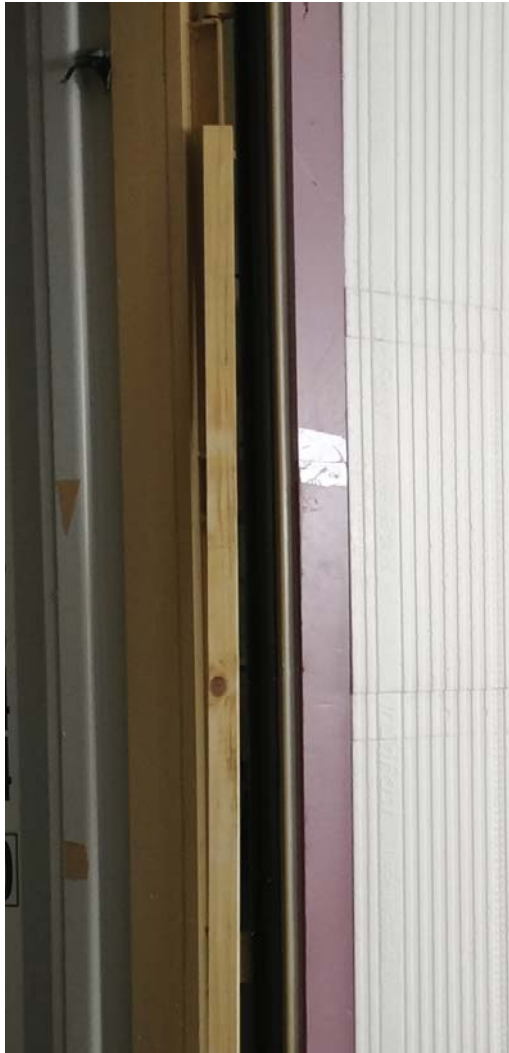
The pink foam is kept back to allow for the trim piece.
