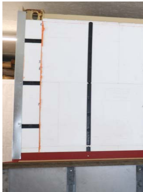
Metal flashing installed for added attachment.
