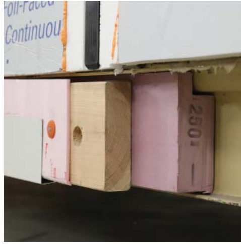
Option one for insulating and furring out the beam.
