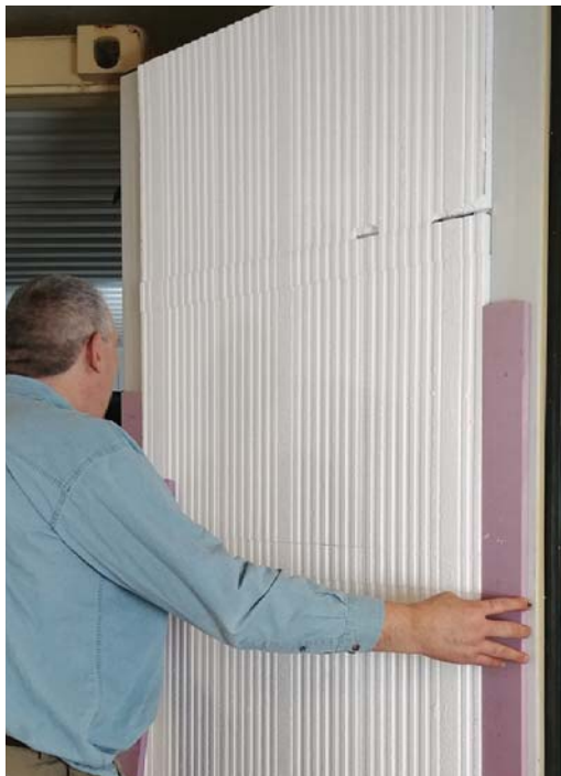
3/4" foam on the vertical rails.
