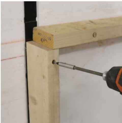
Screw framing into InSoFast stud.
