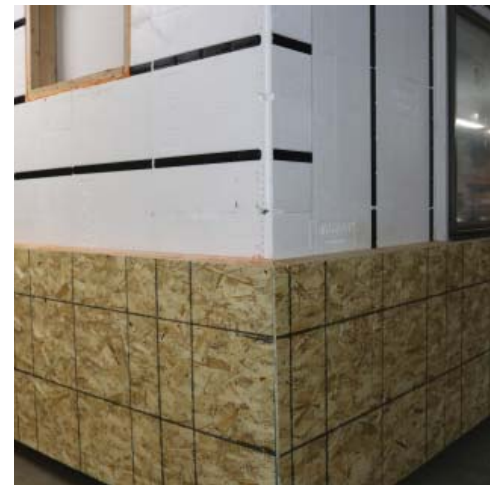
Exterior build out is ready for WRB.
