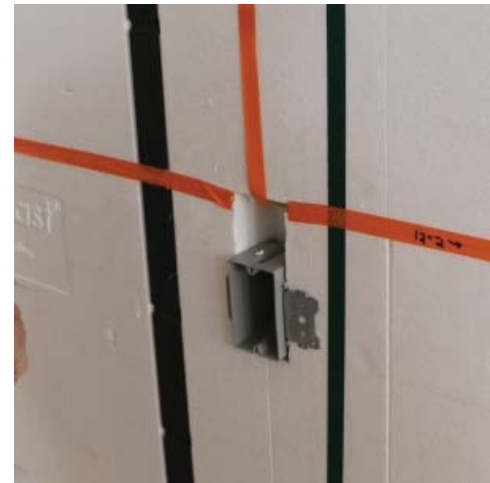
Foam in box after wiring has been run.
