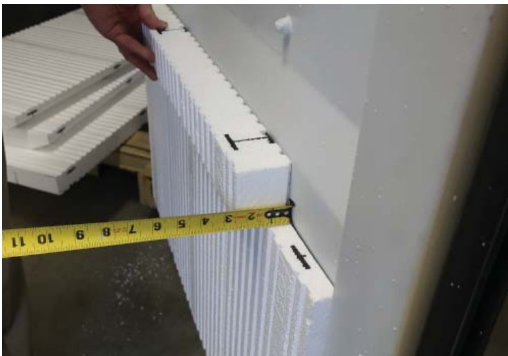
Measure for the thickness needed.
