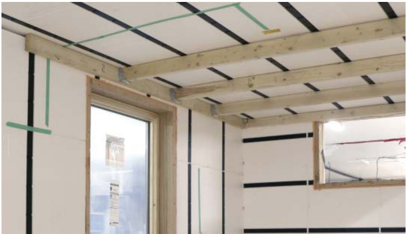
2x4 framework for allows for additional insulation.
