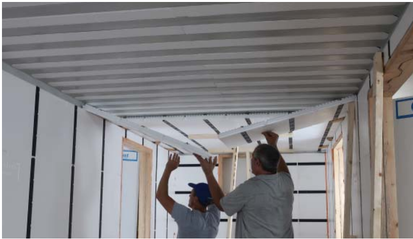
Installing the ceiling panels.
