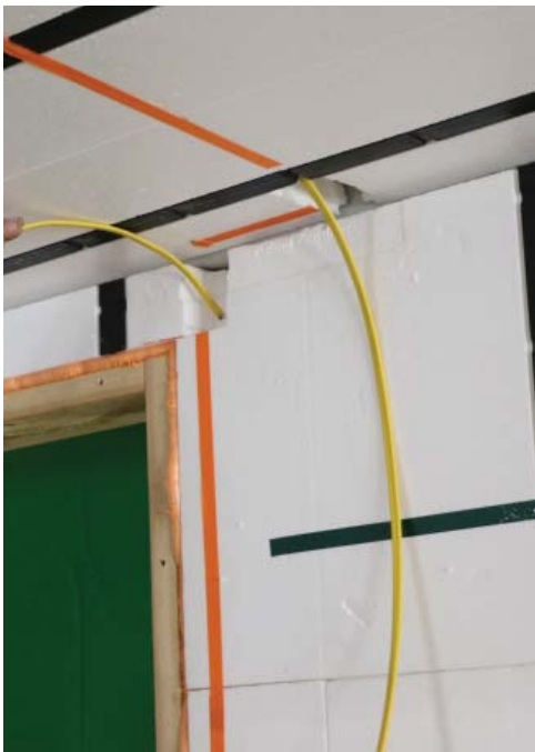
Running wiring down the wall.
