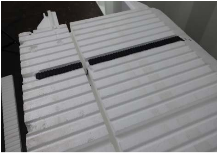
Foam is removed to accommodate the rail.
