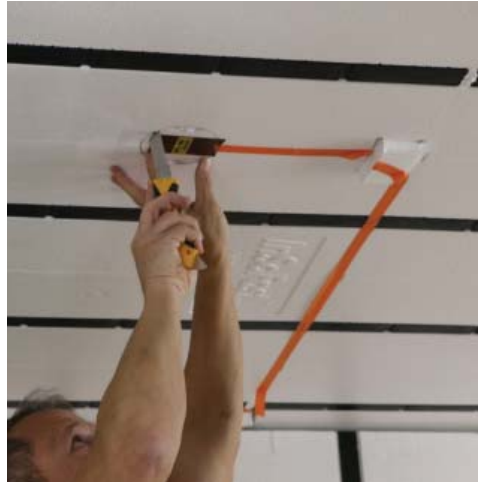
Cutting out for round outlet box.
