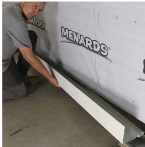
Bottom flashing installed over the WRB.
