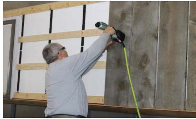
Vertical siding is nailed to wood furring strips.
