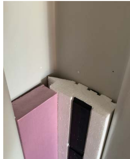
Corner detail for LowPro. Spray foam gaps.
