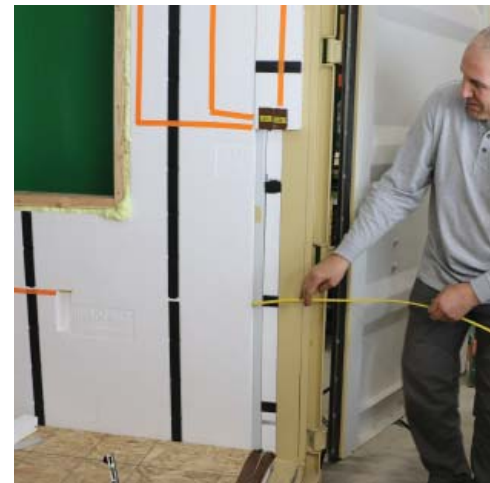
Wire in horizontal raceway.
