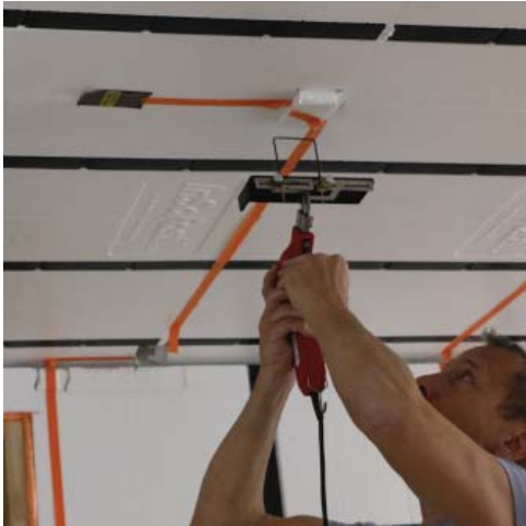
Cutting out raceway intersection.
