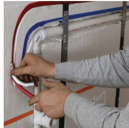
Install bend supports.
