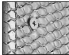
Wire lath to steel or wood studs.
