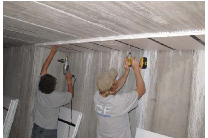
Panels installed with Tapcon screws.
