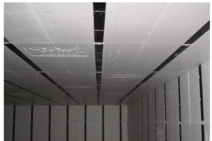
Ready for drywall.
