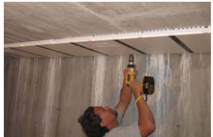
Panels installed with Tapcon screws.
