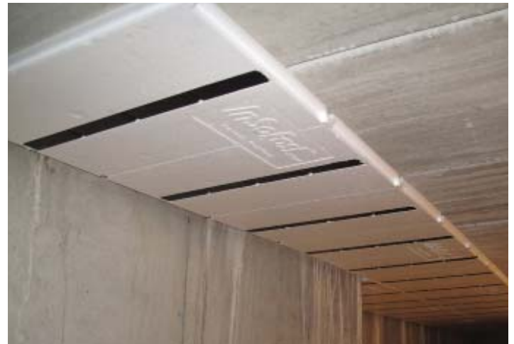
Install ceiling panels first.
