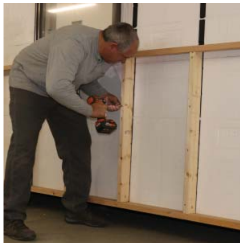
Boxing out the low part of the exterior.
