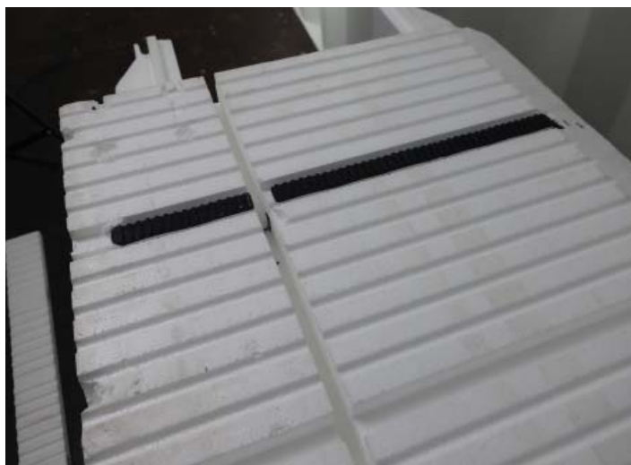
Foam is removed to accommodate the rail.
