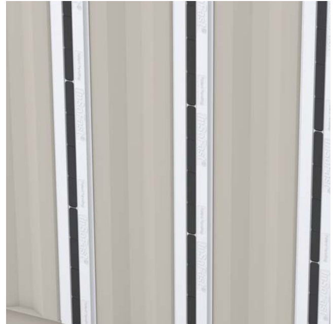
Install the LowPro Inserts in the corrugations.
