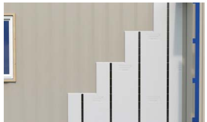
Install the panels in a running bond pattern.
