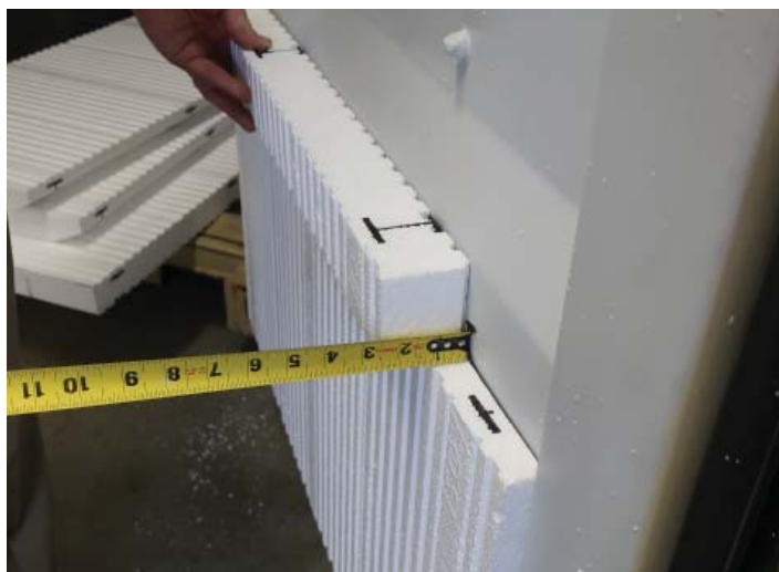
Measure for the thickness needed.
