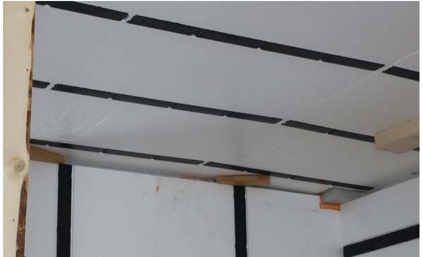
Install blocks or shims to hold panel in place around perimeter.
