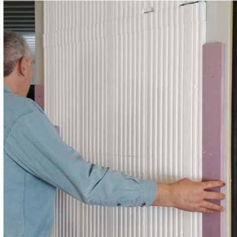
3/4" foam on the vertical rails.
