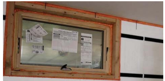
When fitting panels around openings, leave a 1/4" gap for spray foam.
