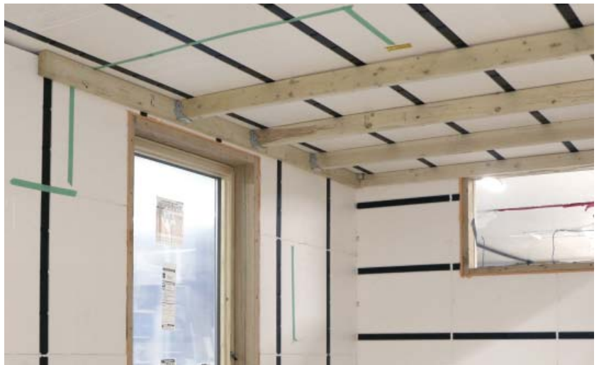
2x4 framework for allows for additional insulation.
