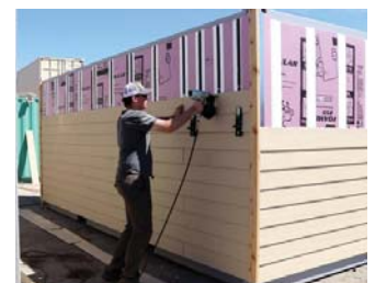
Exterior Siding Pages 22-23
