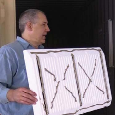
Use plenty of adhesive on the doors.
