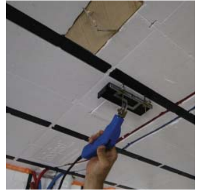
Use a hot knife to cut out for 1x3.
