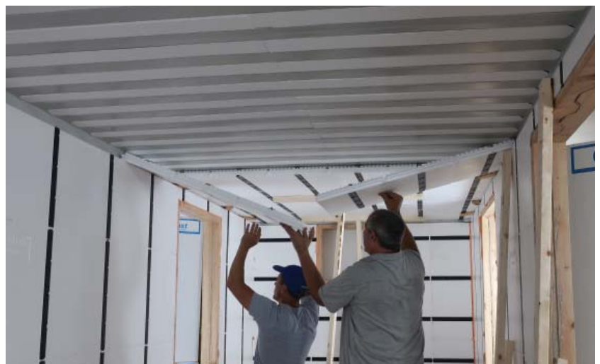
Installing the ceiling panels.
