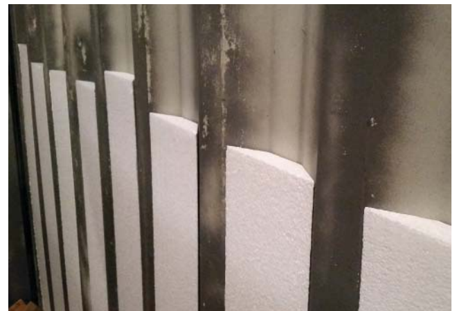
Installing side wall inserts.
