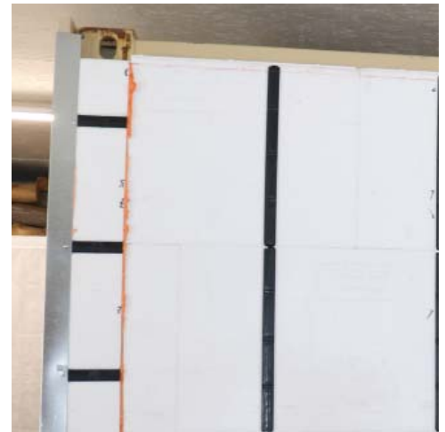
Metal flashing installed for added attachment.
