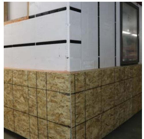
Exterior build out is ready for WRB.
