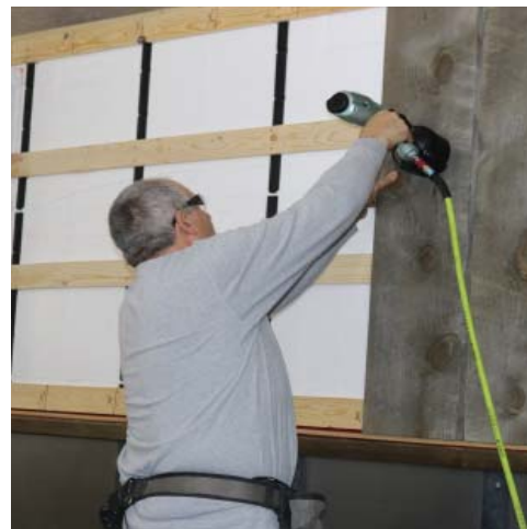
Vertical siding is nailed to wood furring strips.
