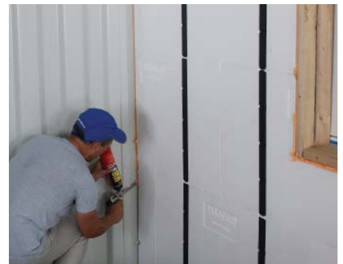
Spray foam in corners to prevent air movement.
