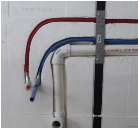
Use protection plates where necessary.
