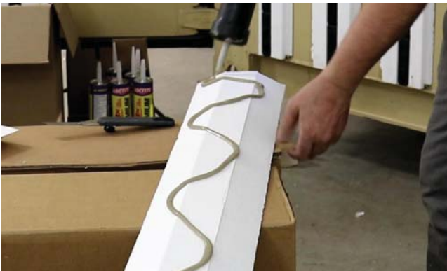
Applying adhesive to side wall insert.
