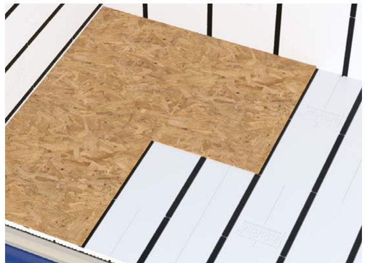
Make sure the long seam of the plywood does not line up with the InSoFast panels.
