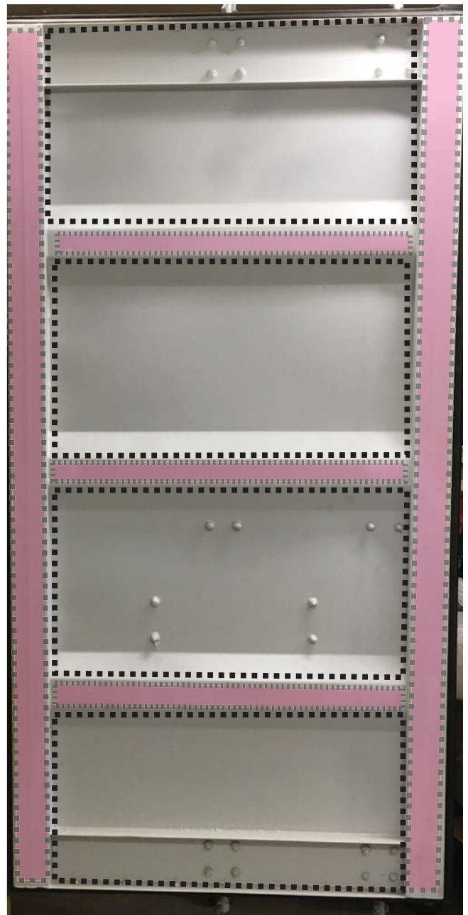
InSoFast is used for the middle and sheet foam for the pink areas.
