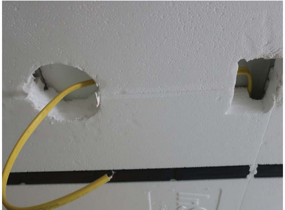
Running wire around the corner requires an access hole.
