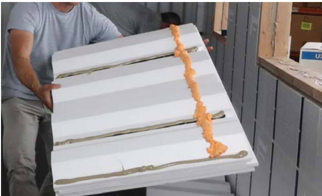
Adhesive and spray foam on CX panels.
