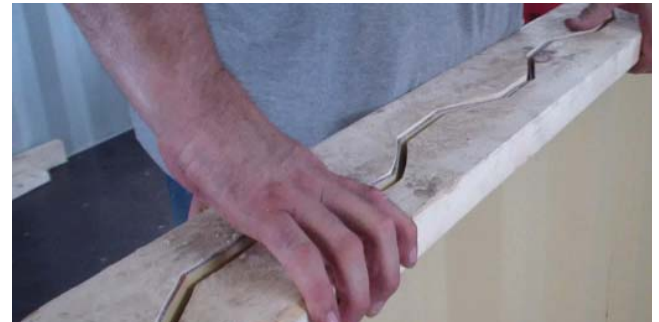
Wood jamb is cut to fit the corrugations.
