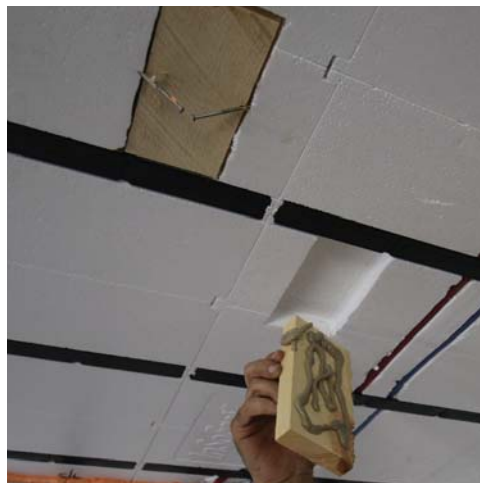
Use PL Premium to glue the blocks in place.
