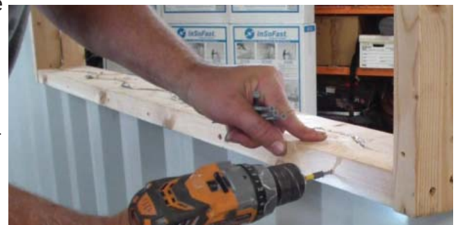
Wood jamb installed.
