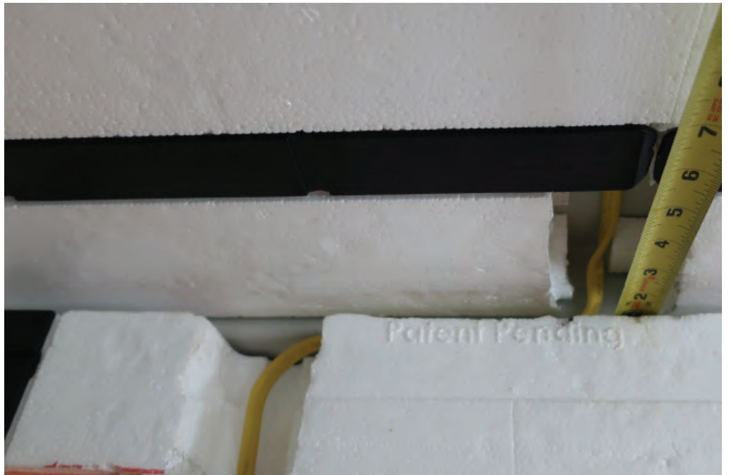
Push with wiring all the way back to the beam.
