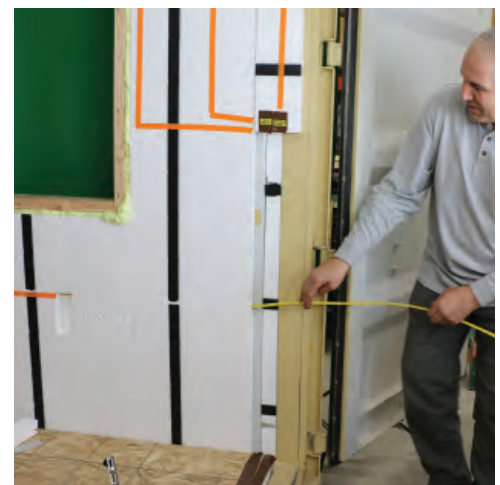
Wire in horizontal raceway.
