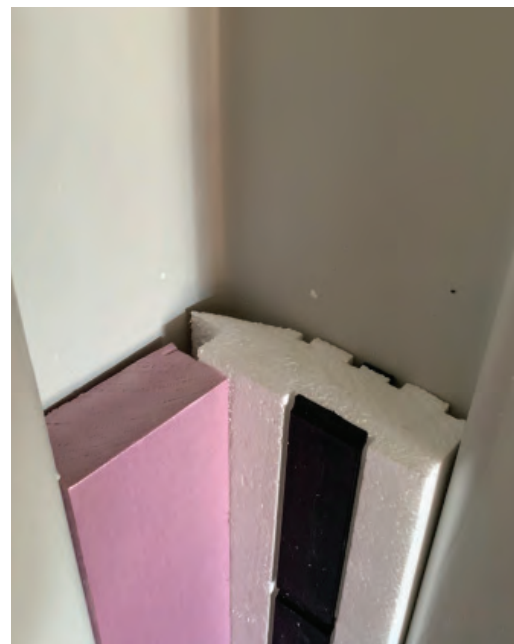
Corner detail for LowPro. Spray foam gaps.
