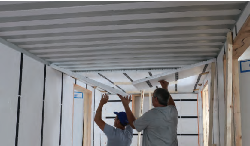
Installing the ceiling panels.
