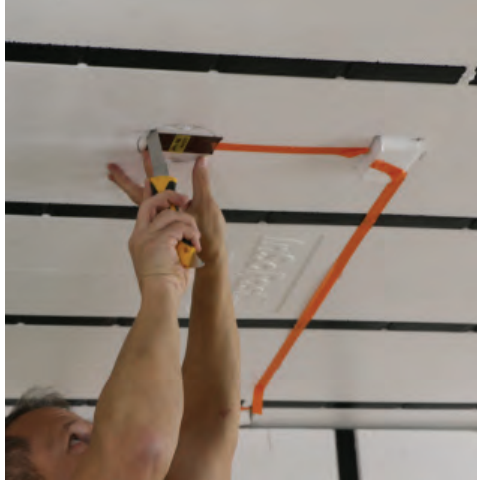
Cutting out for round outlet box.
