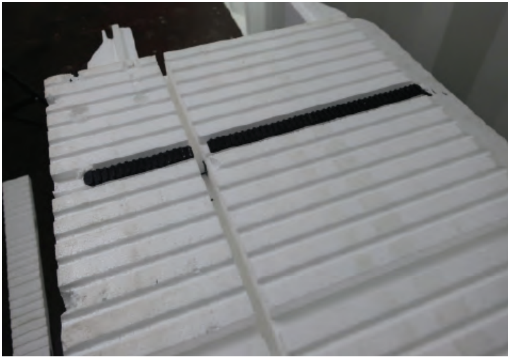
Foam is removed to accommodate the rail.
