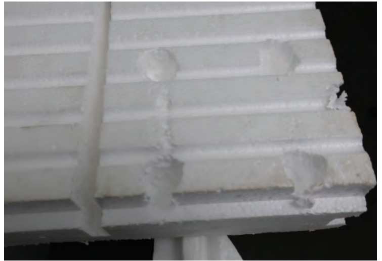
Drill out the foam where the fastener heads are located.
