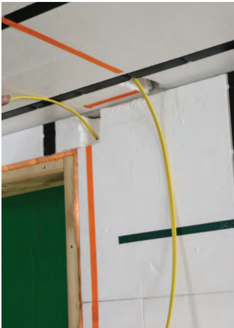
Running wiring down the wall.
