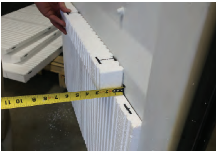
Measure for the thickness needed.
