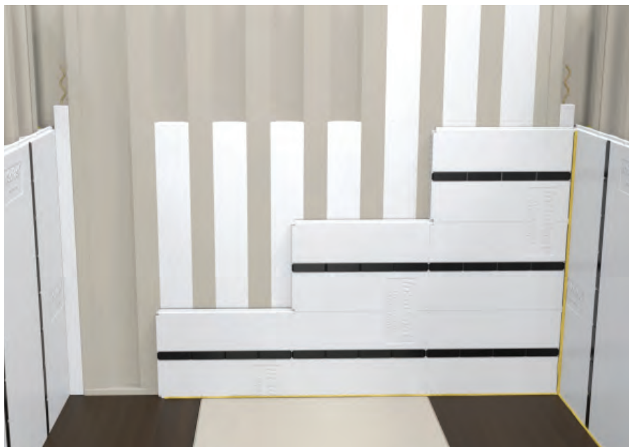
Finish installing inserts and panels on the end wall.
