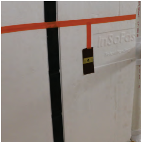
Outlet located below horizontal raceway.
