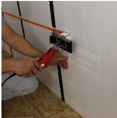
Cutting out using hot knife with sled attachment.
