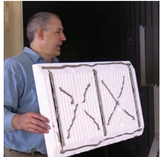
Use plenty of adhesive on the doors.
