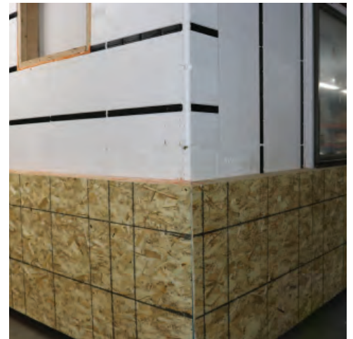
Exterior build out is ready for WRB.
