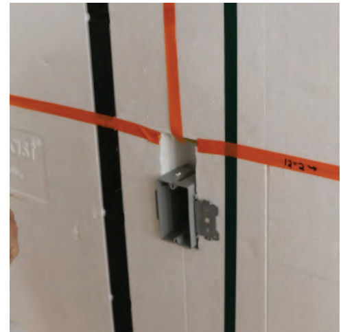
Foam in box after wiring has been run.
