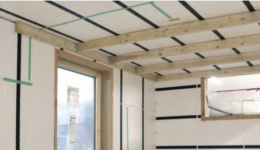
2x4 framework for allows for additional insulation.
