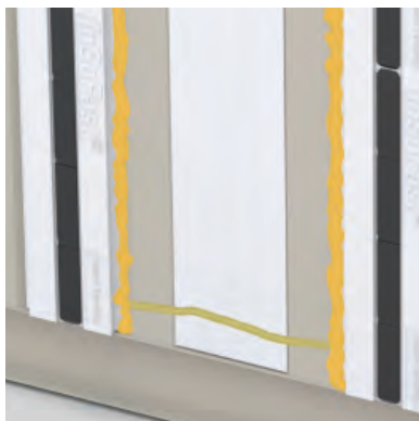
Omit spray foam at bottom for drainage.
