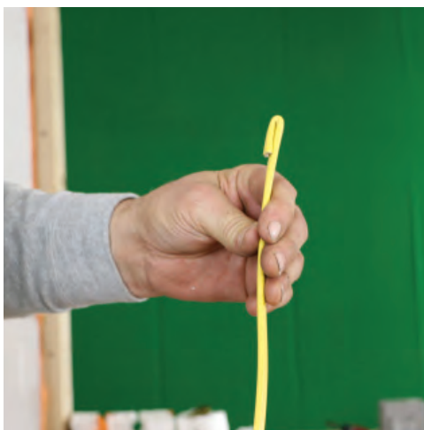
Bend over the tip of with wire when pushing through.
