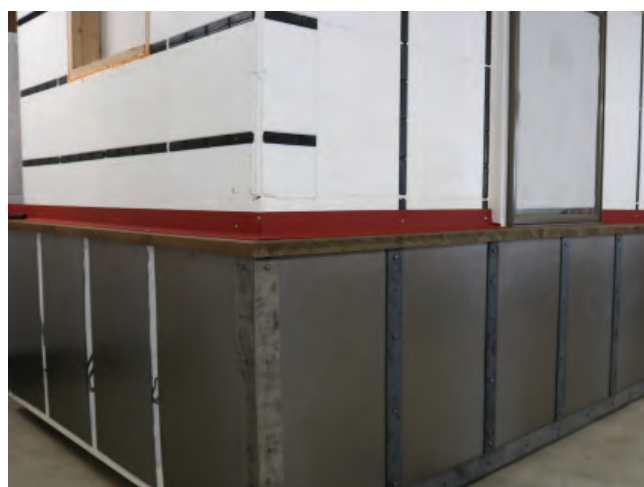
Raw steel was added on lower part of wall.
