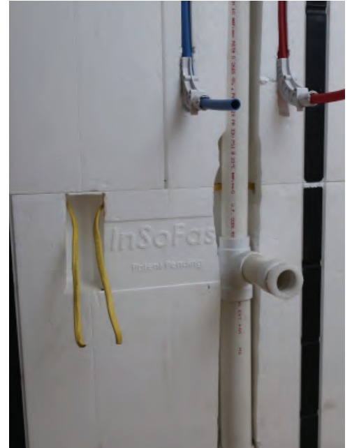
The CX 44 panel can accommodate a 2" PVC pipe.
