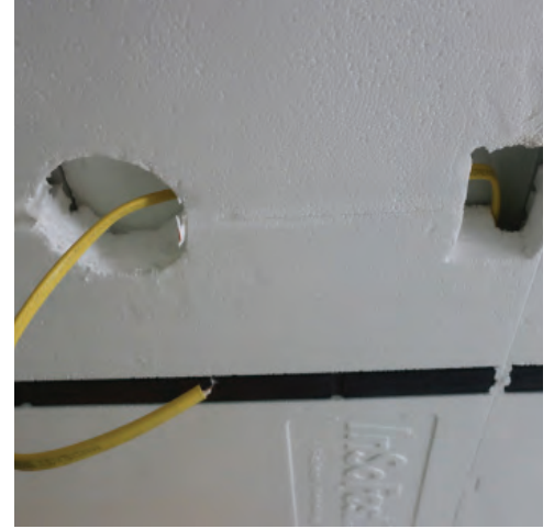
Run wire around the corner.
