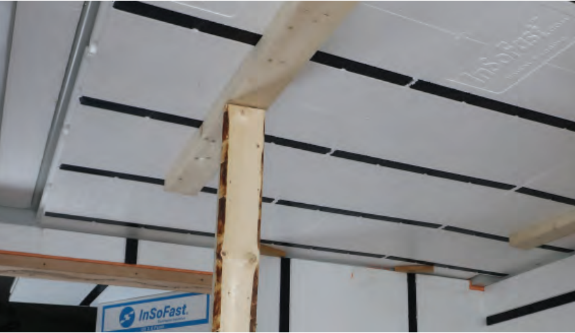
Installing blocks to hold panel in place around perimeter.
