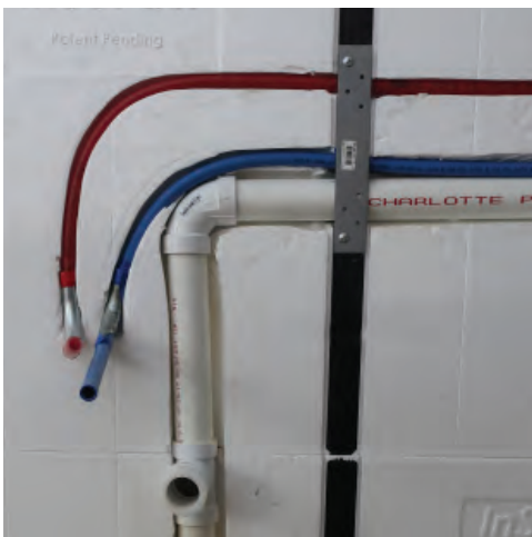
Use protection plates where necessary.
