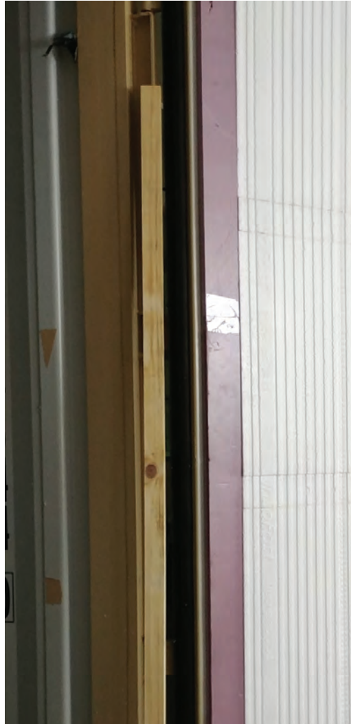
The pink foam is kept back to allow for the trim piece.
