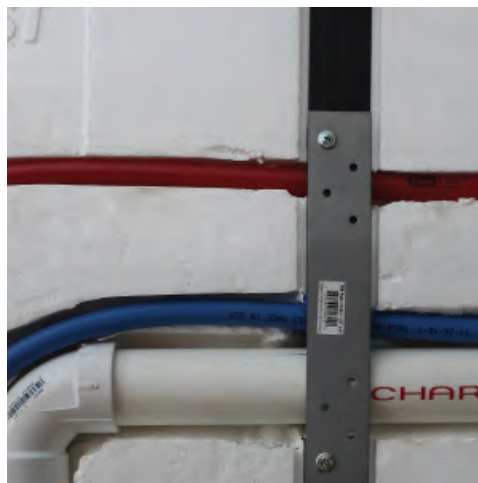
Pex pipe running along side waste.
