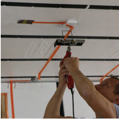
Cutting out raceway intersection.
