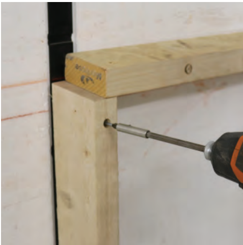
Screw framing into InSoFast stud.
