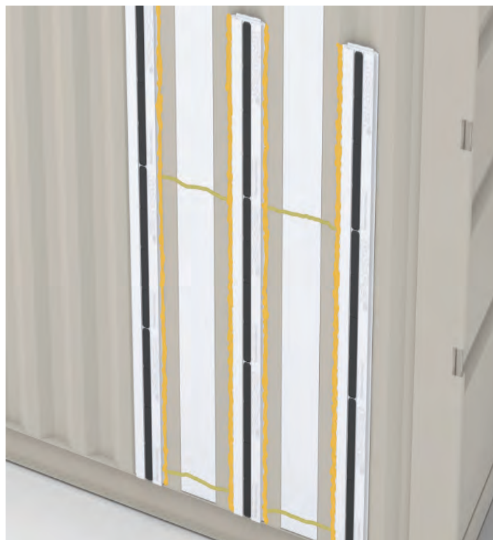
Place PL Premium horizontally and spray foam along the edges.
