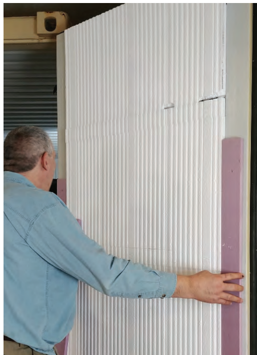
3/4" foam on the vertical rails.
