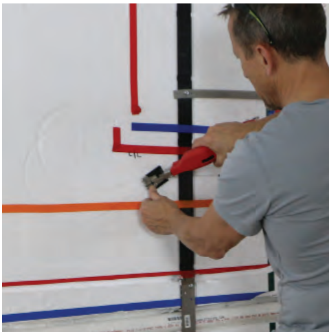
Use hot knife to cut out for pex pipe.
