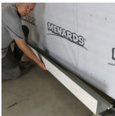
Bottom flashing installed over the WRB.
