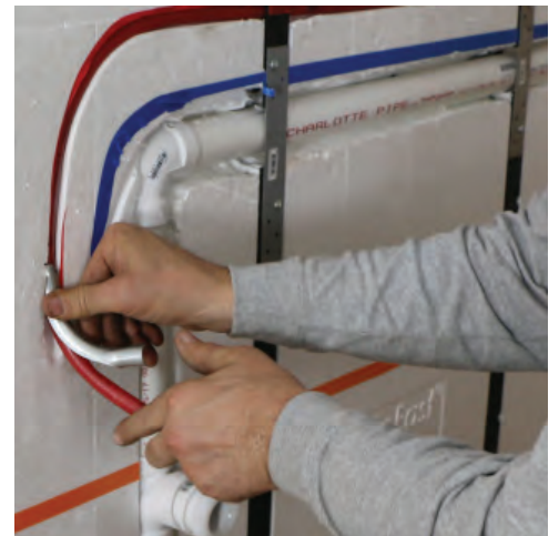
Install bend supports.
