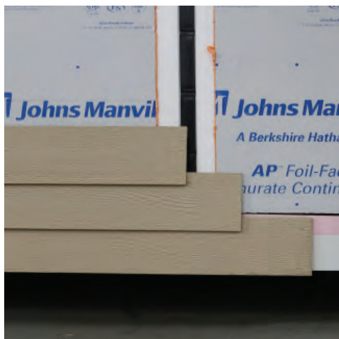
Nail or screw on horizontal siding.
