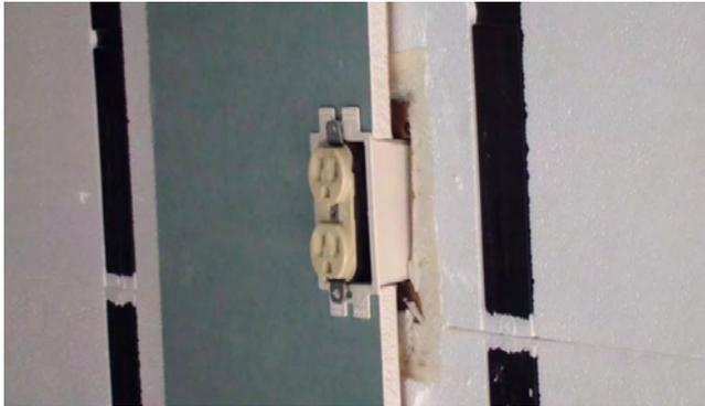
17. Completed extension box with a cut-away drywall cross section
