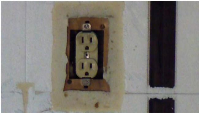
14. Spray foaming completely around the outlet provides an air and moisture barrier that will protect the electrical box.
