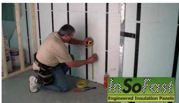
2. Measure mark and locate where you want your electrical box to be installed. Next press the outlet box against the foam to create a mark or an outline to guide you in cutting out for the electrical box.
