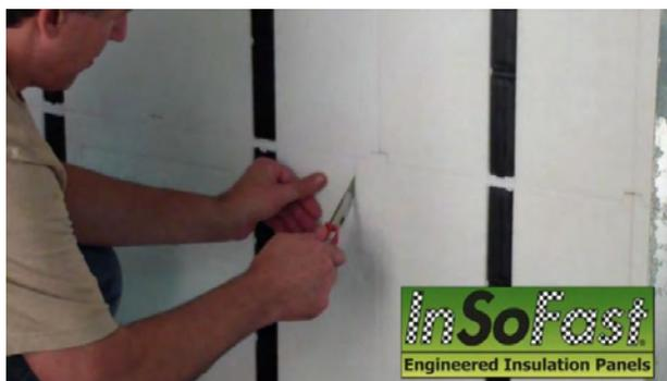
3. Then slice the foam like you are cutting a loaf of bread. It is okay to cut out a larger opening than the electrical box. You will need room to be able to work with the wiring.
