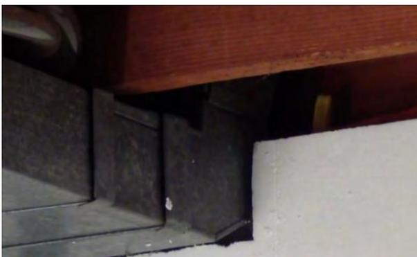
8. InSoFast raceways are at 1 1/4" deep and meet the electrical code. Standard Romex type wiring or Flexible conduit can also be used please consult with your local electrical inspector.
