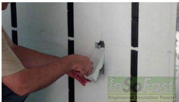
4. Once we cut the out for the opening to the depth we need pop out the piece of foam you just cut. You can save this piece of foam to reinsert later or spray foam and seal the area.
