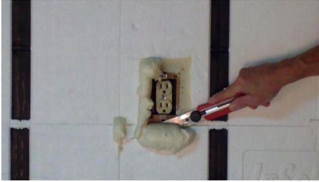
13. After the spray foam cures you will be able to go back and trim away the excess foam with a razor blade knife.
