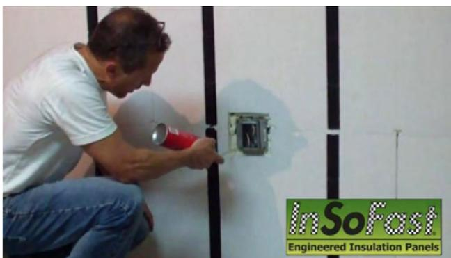
12. Here we are demonstrating the use of spray foam to seal air seal the box to the wall. Spray foaming completely around the outlet provides an air and moisture barrier that will protect the electrical box.
