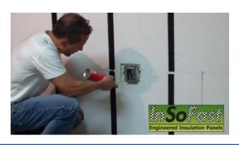
12. Here we are demonstrating the use of spray foam to seal air seal the box to the wall. Spray foaming completely around the outlet provides an air and moisture barrier that will protect the electrical box.
