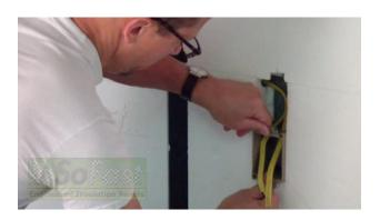
11. Secure the box to the wall by either a concrete fastener or spray foam adhesive always check with the building codes to what they require.
