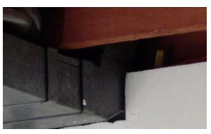
8. InSoFast raceways are at 1 1/4" deep and meet the electrical code. Standard Romex type wiring or Flexible conduit can also be used please consult with your local electrical inspector.
