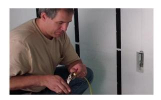
5. Pulling wires through InSoFast is easy! Make sure your wire is not kinked. Bend the leading edge of the wire with a linemen's pliers so it does not catch in the channel's raceway.
