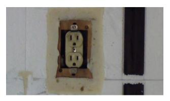
14. Spray foaming completely around the outlet provides an air and moisture barrier that will protect the electrical box.
