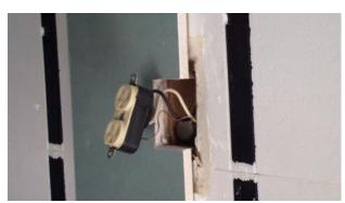
15. Once the drywall is installed over the InSoFast you may find that the electrical box is ½" to deep. This can be easily fixed.
