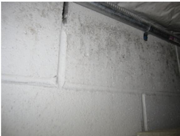
**Figure 1-2** Mold growth on painted concrete masonry. The cool masonry wall separates a classroom from an ice rink. Humid air in the classroom provides moisture that condenses on the painted surface of the masonry. That moisture allows mold to grow on the paint film.
