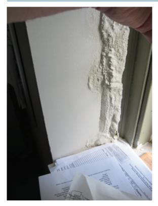
**Figure 1-10** Further rain damage to interior plaster. At another location on an office window in the building shown in Figure 1-8, rain seepage turns gypsum board joint compound to a fluid, causing the gypsum to bubble and lift.
