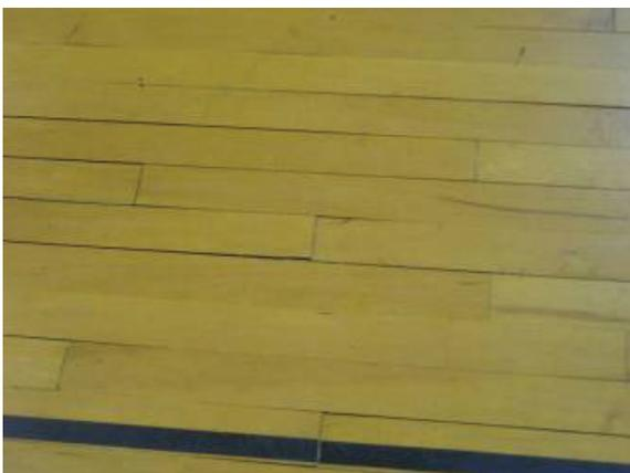
**Figure 1-12** Hardwood gymnasium floor warped by moisture in the cavity below it. Water rises through the concrete sub-floor. The source of the moisture is rainwater that has not been drained away from the foundation of the building.
