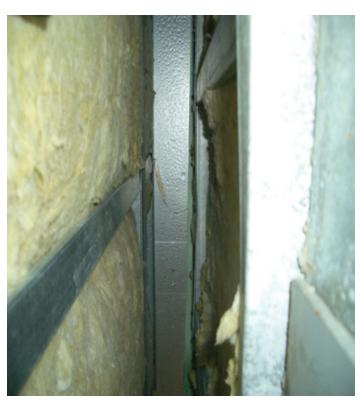
Condensation occurs on a C-channel at the top of a parapet wall located in a cold climate. The building is humidified and pressurized with filtered outdoor air to maintain specified interior conditions.
