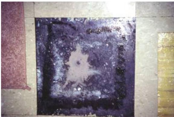
**Figure 1-13** Tile adhesive that failed to cure because of water in the concrete and high pH. The tile can be removed by hand. The floor is a concrete slab-on-grade. The water visible in the photo evaporates into the room after several minutes. Its source may be liquid water wicking up from the sub-slab fill or water vapor migrating through the slab.
