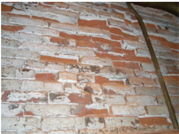
**Figure 1-14** Damage to bricks caused by the migration of soluble salt through them. Salts in the brick or mortar dissolve in rainwater that wicks through the brick. The water evaporates in the building's interior, and the salt left behind crystalizes and splits the surface layer off the brick, exposing its interior. This process is called sub-fluorescence.
