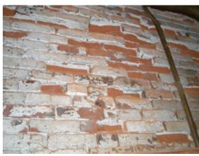
**Figure 1-14** Damage to bricks caused by the migration of soluble salt through them. Salts in the brick or mortar dissolve in rainwater that wicks through the brick. The water evaporates in the building's interior, and the salt left behind crystalizes and splits the surface layer off the brick, exposing its interior. This process is called sub-fluorescence.
