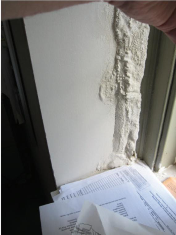
**Figure 1-10** Further rain damage to interior plaster. At another location on an office window in the building shown in Figure 1-8, rain seepage turns gypsum board joint compound to a fluid, causing the gypsum to bubble and lift.
