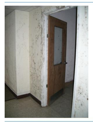
**Figure 1-1** Mold growing on the surface of painted gypsum board and trim. Long-term high humidity is the source of the moisture that allowed the mold growth. All of the walls experienced similar near-condensation conditions. Consequently, the mold growth is widespread rather than concentrated in a single damp area.
