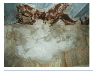
**Figure 1-4** Corrosion of galvanized fluted steel floor deck. The floor is at grade level. The source of the water is rainwater seepage.
