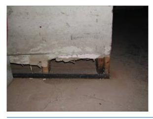
**Figure 1-11** Gypsum board on the lower edge of a basement wall dissolved by seasonal flood waters. The water table is just below the basement floor during dry weather and rises several inches above the floor during heavy spring rains.
