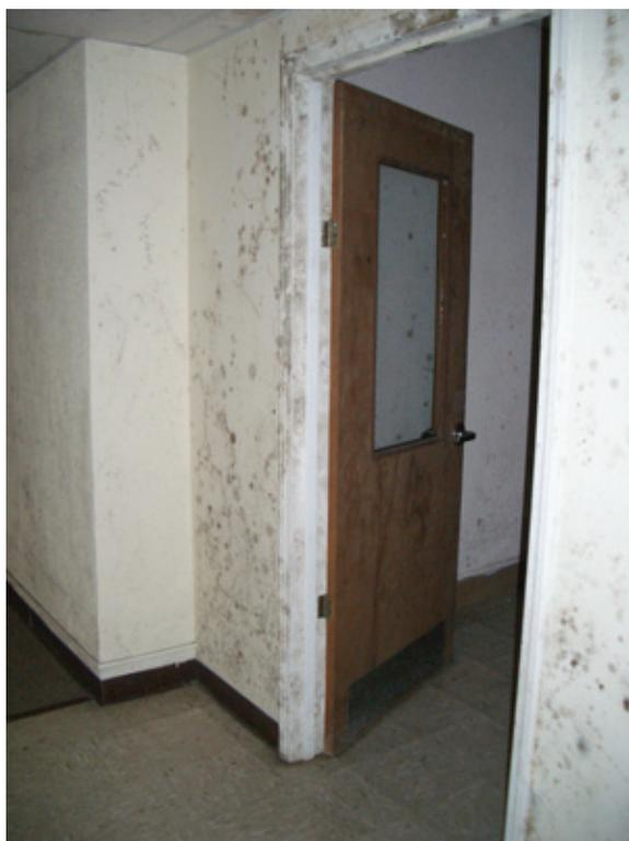
**Figure 1-1** Mold growing on the surface of painted gypsum board and trim. Long-term high humidity is the source of the moisture that allowed the mold growth. All of the walls experienced similar near-condensation conditions. Consequently, the mold growth is widespread rather than concentrated in a single damp area.
