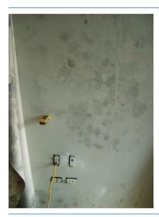
**Figure 1-7** Condensation behind vinyl wallpaper in a warm, humid climate. Condensation and mold growth occurs behind the vinyl wallpaper on both exterior and interior walls. Air leaks in the return plenum of the air handler depressurizes the interior and exterior wall cavities. Warm, humid exterior air is drawn from outside through air leaks in a heavy masonry wall.
