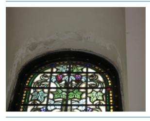
**Figure 1-9** Interior plaster damaged by rain seeping around a window in a brick building. The inside of the exterior wall is insulated with closed-cell spray foam. Consequently, the wall cannot dry to the interior, so it retains excessive amounts of moisture. At the point where the plaster on the window return meets the brick wall, rainwater wicks into the plaster causing the damage seen in this photo.
