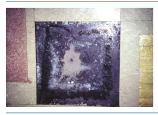
**Figure 1-13** Tile adhesive that failed to cure because of water in the concrete and high pH. The tile can be removed by hand. The floor is a concrete slabon-grade. The water visible in the photo evaporates into the room after several minutes. Its source may be liquid water wicking up from the sub-slab fill or water vapor migrating through the slab.
