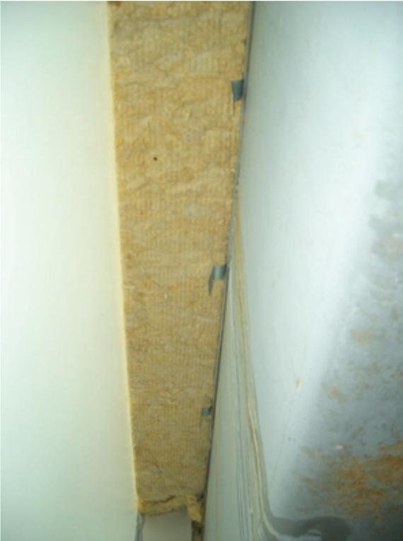
**Figure 1-5** Corrosion of structural steel in a ceiling cavity in a cold climate. The steel extends into the exterior wall assembly. During cold weather, the steel near the wall is chilled by cold outdoor air. The building is humidified, and condensation from high indoor humidity provides the moisture that rusts the cold steel.
