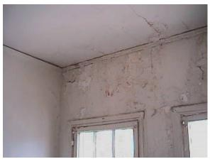
**Figure 1-8** Rainwater leaks in a rooftop parapet wall result in damaged plaster and peeling paint. Rainwater is drawn into this brick assembly by capillary action, and the moisture is aided in its downward migration by gravity. The peeling paint contains lead and results in an environmental hazard as well as physical damage to the plaster.
