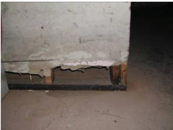
**Figure 1-11** Gypsum board on the lower edge of a basement wall dissolved by seasonal flood waters. The water table is just below the basement floor during dry weather and rises several inches above the floor during heavy spring rains.
