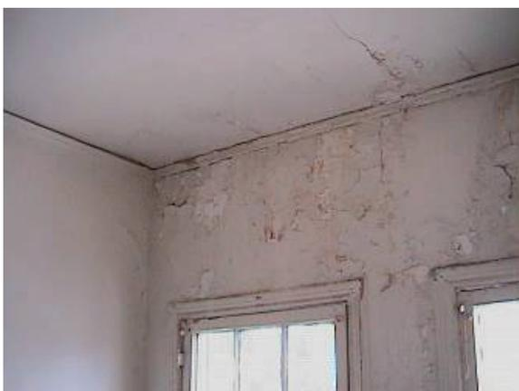
**Figure 1-8** Rainwater leaks in a rooftop parapet wall result in damaged plaster and peeling paint. Rainwater is drawn into this brick assembly by capillary action, and the moisture is aided in its downward migration by gravity. The peeling paint contains lead and results in an environmental hazard as well as physical damage to the plaster.
