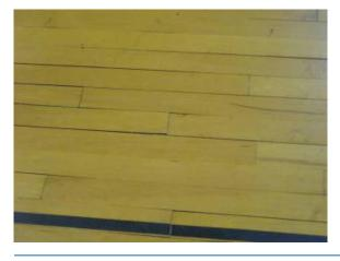
**Figure 1-12** Hardwood gymnasium floor warped by moisture in the cavity below it. Water rises through the concrete sub-floor. The source of the moisture is rainwater that has not been drained away from the foundation of the building.
