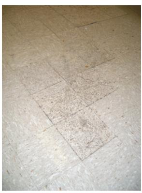
**Figure 1-3** Mold growth on vinyl floor tile. Long-term high humidity provided moisture that was absorbed into the cool vinyl tile and supported mold growth. Also note that the high humidity caused the adhesive attaching the tile to the floor to fail, allowing the tile to become loose.
