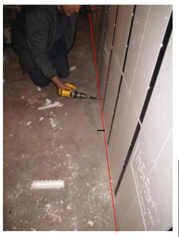
Slowly turn the screw in until the wall is level with the chalk line. Repeat until the entire base of the wall has been trued to the line.
