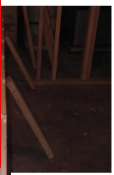
Although it is hard to see, the 4" set screw is holding the panel away from the wall keeping the InSoFast panel plumb.
