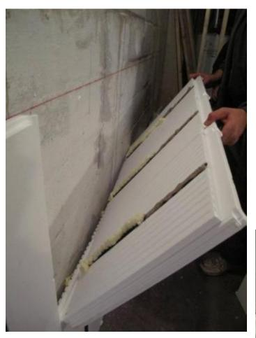
Note the 2 different adhesives being used to provide proper glue contact to secure the panel to the wall.
