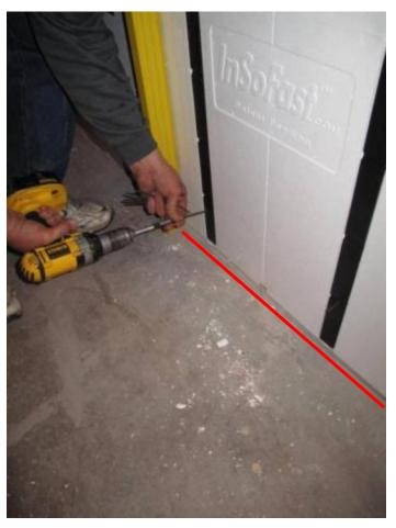
Use 4" deck or drywall screws. Screw through the panel's stud until fastener comes in contact with solid wall. Then slowly screw the fastener in so that the panels are ratcheted out until you meet the chalk line on the floor. Use the chalk line on the floor as a guide to straighten your wall.
