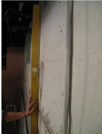
In this photo to the left, if we ignored the bubble and fit our straight edge flush to the top of the wall, the level's straight edge has kicked away from the wall by over 2 ½" at the floor.
