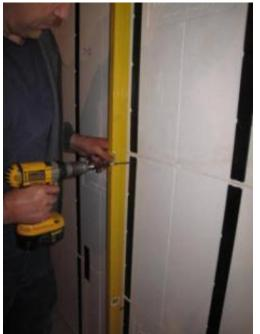
Work your way up the wall. Follow the level using it as a guide and install additional "shim screws" directly above the previous "shim screws" where needed to level out the wall.
