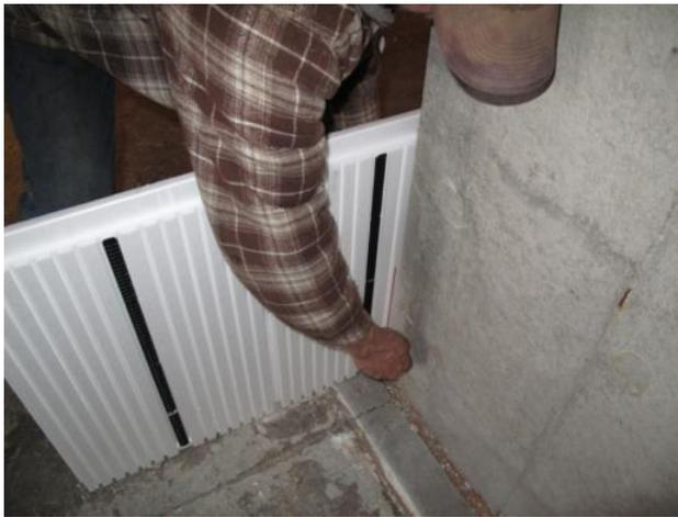
InSoFast is rough framing and not fine carpentry. Cuts should not be tight. You can always go back and fill in any voids or gaps with spray foam.
