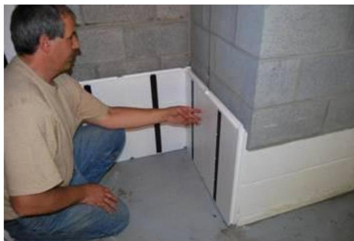
Leaving a  $\frac{1}{4}$ " gap reduces the push out stress on the panels so they remain flat and tight to the wall.
