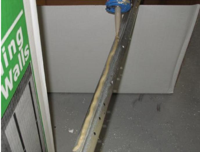
Apply a bead of adhesive directly on to the metal utility corner angle.
