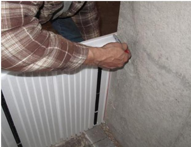
Mark and cut the panels about  $\frac{1}{4}$ " less than actual measurement needed so panels are not tight to the inside or outside corners, leaving a  $\frac{1}{4}$ " gap reduces the push out stress on the panels.
