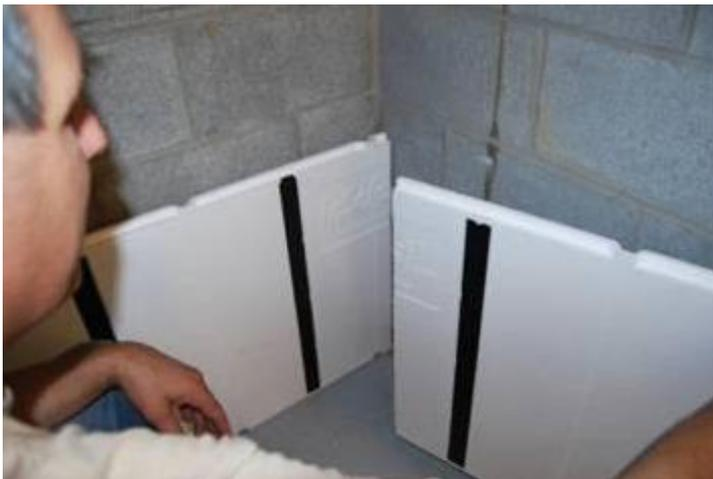
Mark and cut the panels about  $\frac{1}{4}$ " less than actual measurement.
