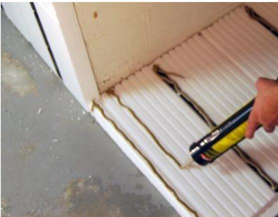
Note the double bead of glue is added at the foam overlap and the concrete wall to assure a nice tight and solid corner. Press into place.
