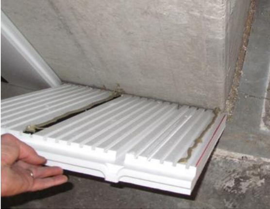
Apply a bead of adhesive directly on to the foam panel at the outside corner's edge and on all studs.
